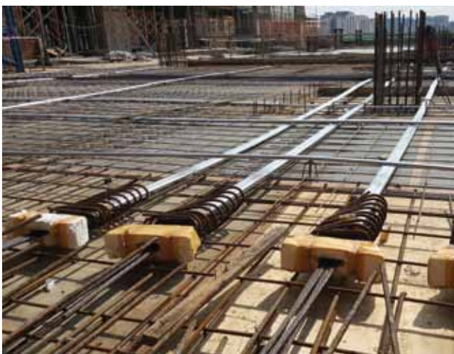
MPT Flat Slab System and flat duct being laid in position.
