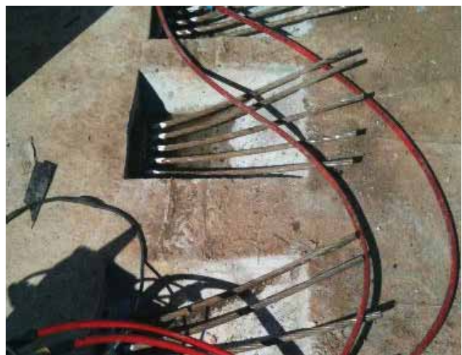
PC strand being marked after stressing.
