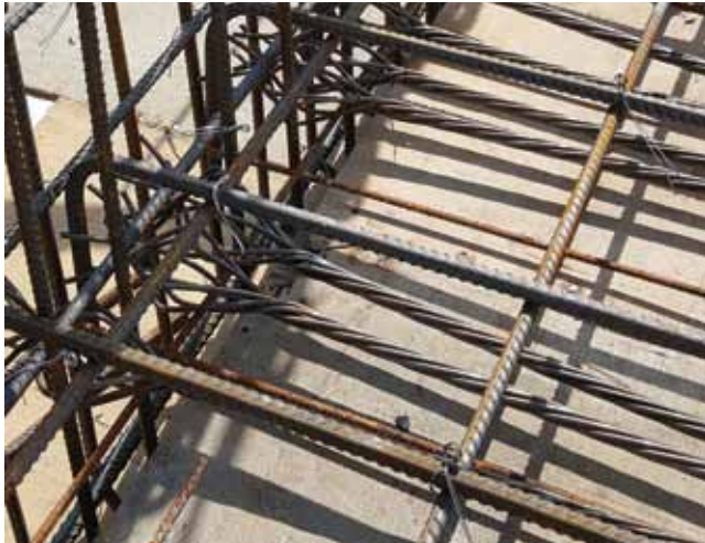
MPT dead end anchorage being laid in position.
