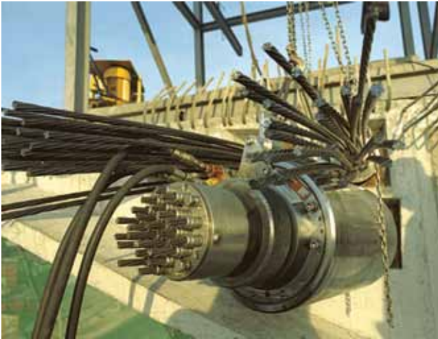
Multi Stressing Jack being hoisted to position.
