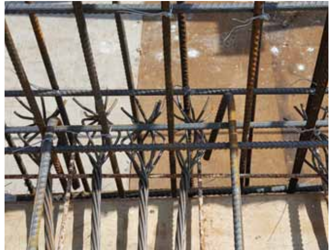
MPT dead end anchorage being laid in position.
